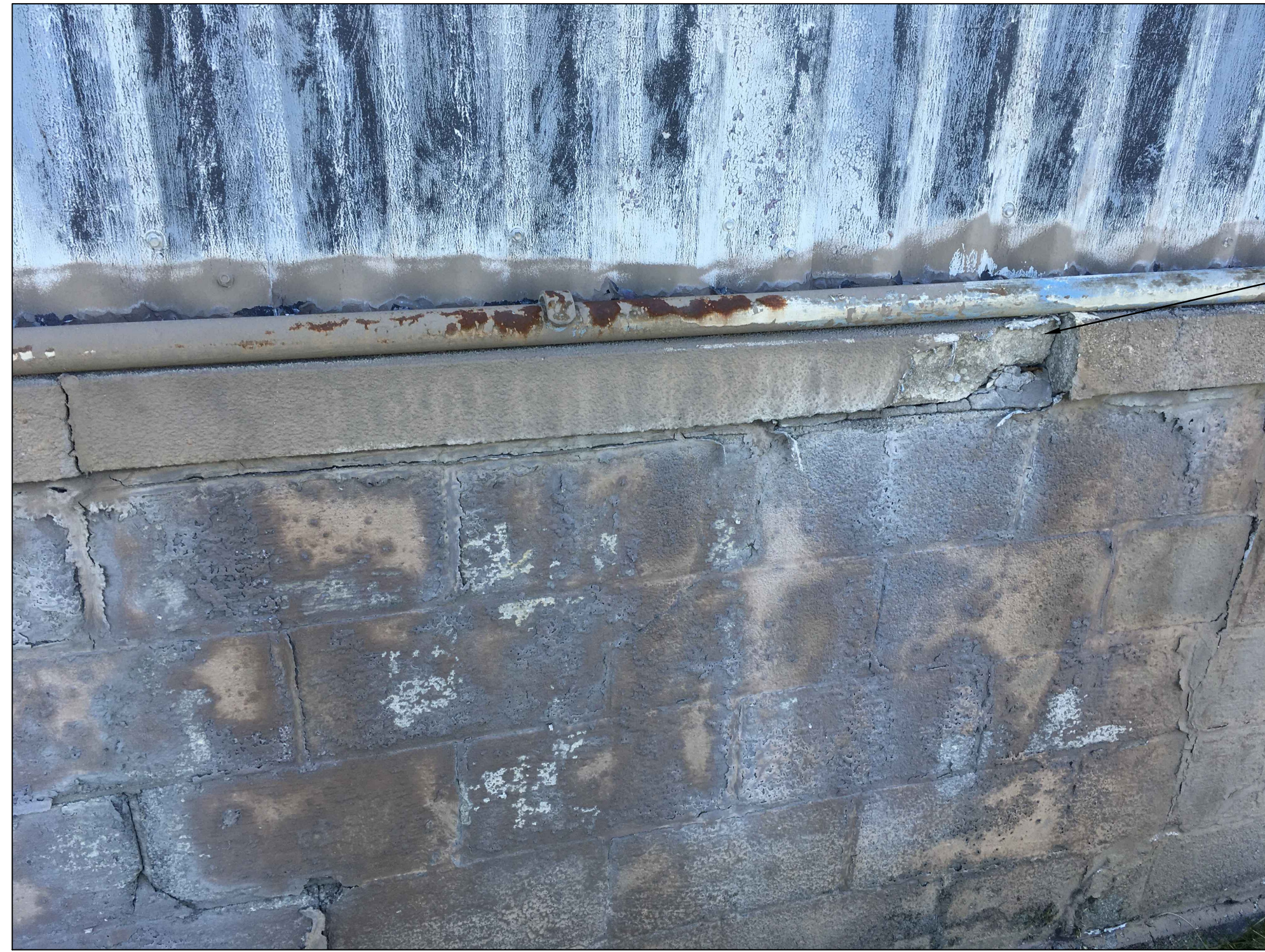
1 TYPICAL BROKEN LINTEL R-101 NOT TO SCALE
